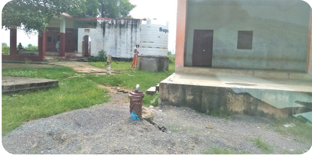
Installation of submersible water pump at nearby villages
